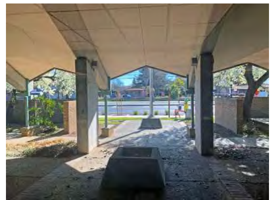
Overhanging eaves facing Folsom Boulevard
